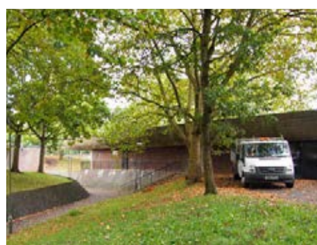
Existing energy centre.
