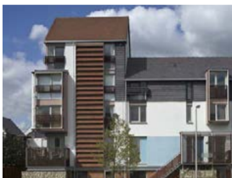
Height and change in material to corner. Abode, Proctor and Matthews
