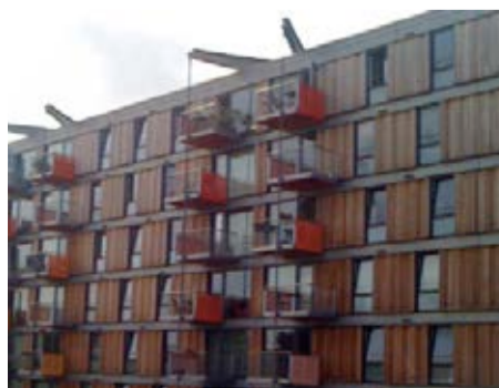
Prominent, lively frontage Adelaide Wharf, Haggerston
