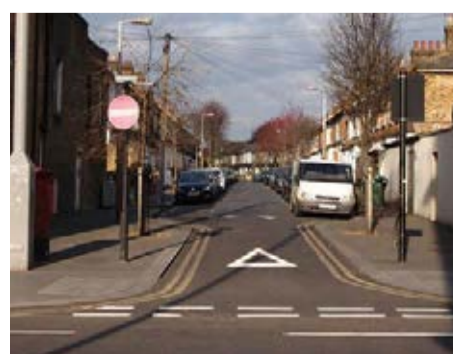
Pinchpoint with access from minor road to more major road, with integrated trees. Leyton.
