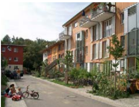
Integrated parking, planting and cycle pedestrian through routes in wide, overlooked shared space., Vauban, Freiburg
