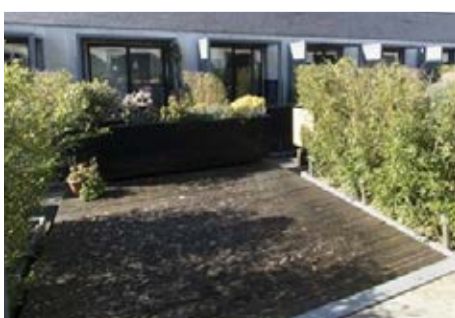
Raised garden decks above parking, with large voids and planting through. Chimney Pot Park.
