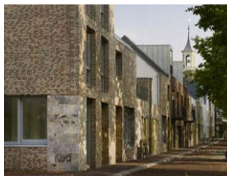
Informal building heights. Molenplien, Netherlands
