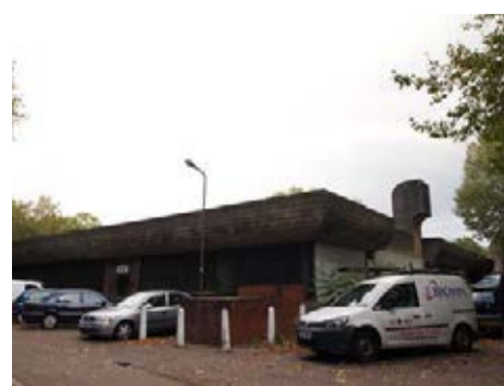
Existing energy centre.
