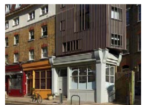
An active ground floor level. Alex Monroe Studios, Southwark
