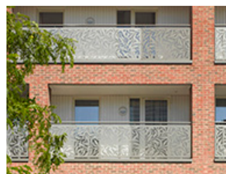
Inset balconies to mid level apartments. Macreanor Lavington
